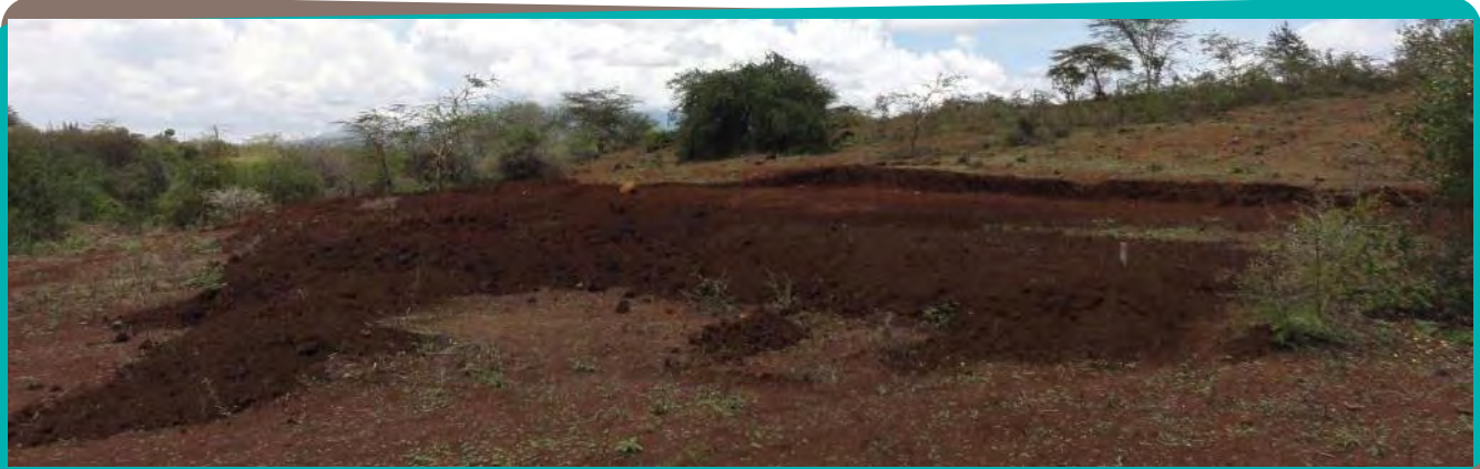
→ The construction site across the river for teacher housing
