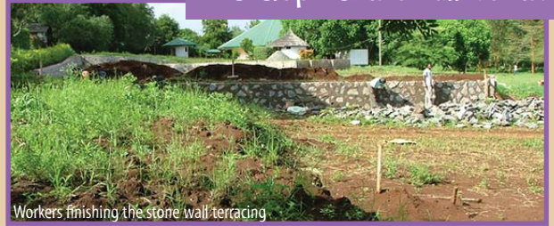
Workers finishing the stone wall terracing
